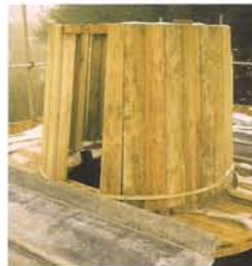
The new tower begins to take shape
